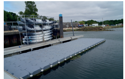
The Saniflos 280 is installed under the pontoon behind the floating buoy
